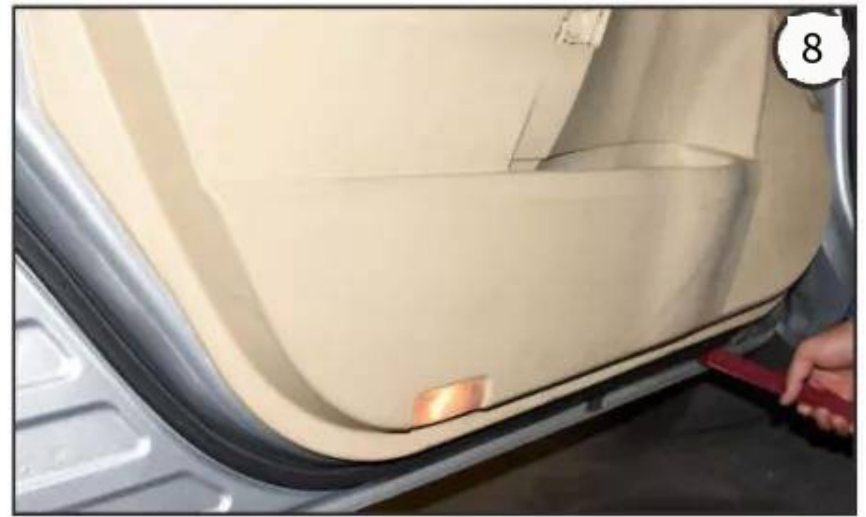
8. Use a pry knife to carefully pry open the peripheral buckle along the edge of the door trim plate, and then remove the door trim plate (FIG. 8)
